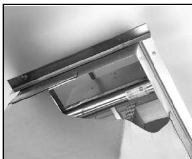
Through Ceiling Membrane Penetration
